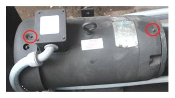
Figure 17. Motor Grease Fittings
