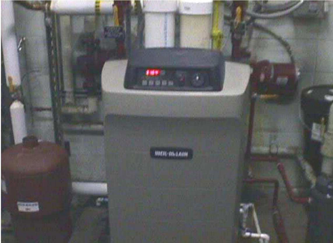
The photo above shows one acceptable alternative for smaller Postal facilities where space is a problem. This is a “Weil McLain Ultra”, high efficient condensing, *cast aluminum*, hot water heating boiler. The vessel itself holds only 1 ½ gallons of water. This unit is a 230,000 btu unit. An optional CSD-1 kit, was also installed with the unit.
